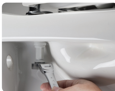
2) Tighten with Spanner
